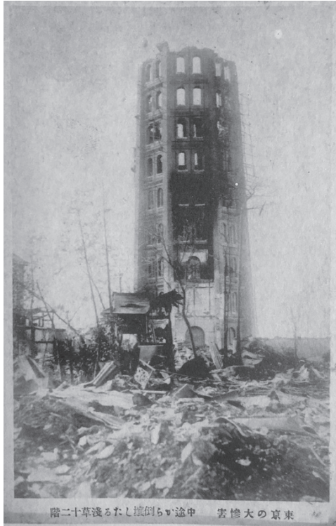
Figure 10: Ryōunkaku: Asakusa Twelve Stories Broken at the Sixth Floor (author's collection)
